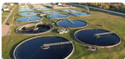
Water, Waste Water Management
